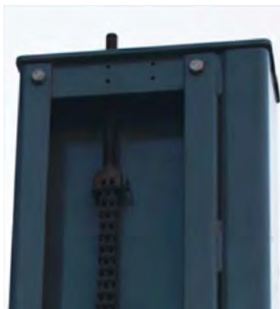
Chart (9) Fixing chain onto top of post
