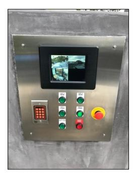
Dimensions: Fascia – 1/8" Thick x 16" Wide x 18-1/8" Tall Box – 6" Deep x 14" Wide x 16-1/8" Tall Location: Outdoors, can be out of sight of the lift Mounting: Recessed wall mounted, anchored inside wall pocket <u>Voltage:</u> 24 VDC <u>Materials:</u> sealant, concrete screws
